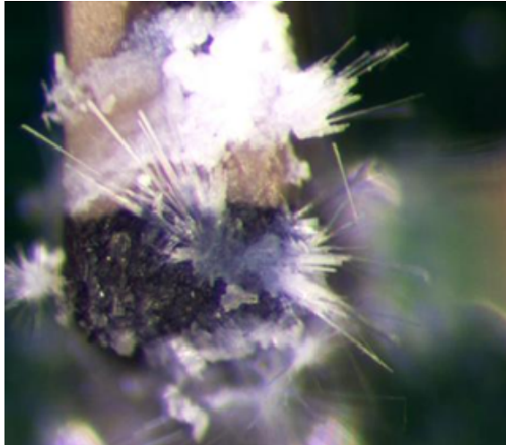
Figure 3 – Capacitor #1 with tin whiskers on power input side
