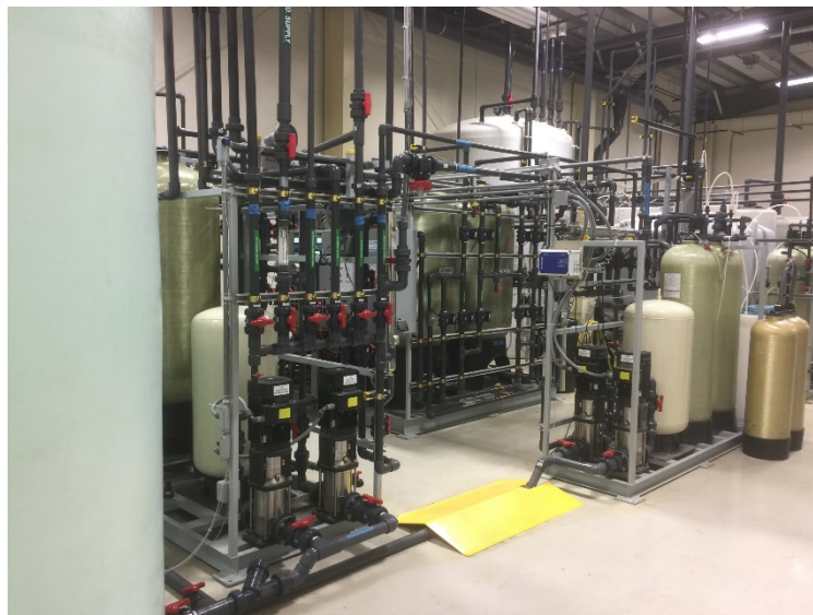
FIGURE 8 – Example of zero liquid discharge system.
